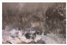
Efflorescence
