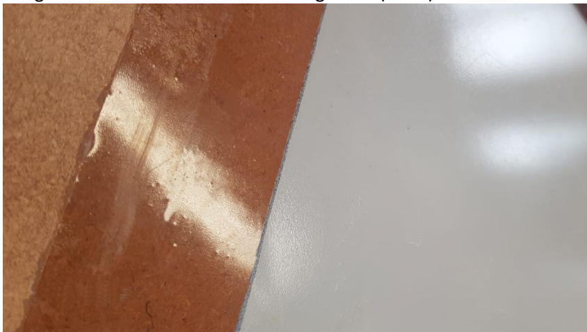
Image of finish – Primer + Self-Leveling finish (1mm)
