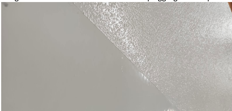
Image of finish – Second coat with anti-slip aggregate if required.
